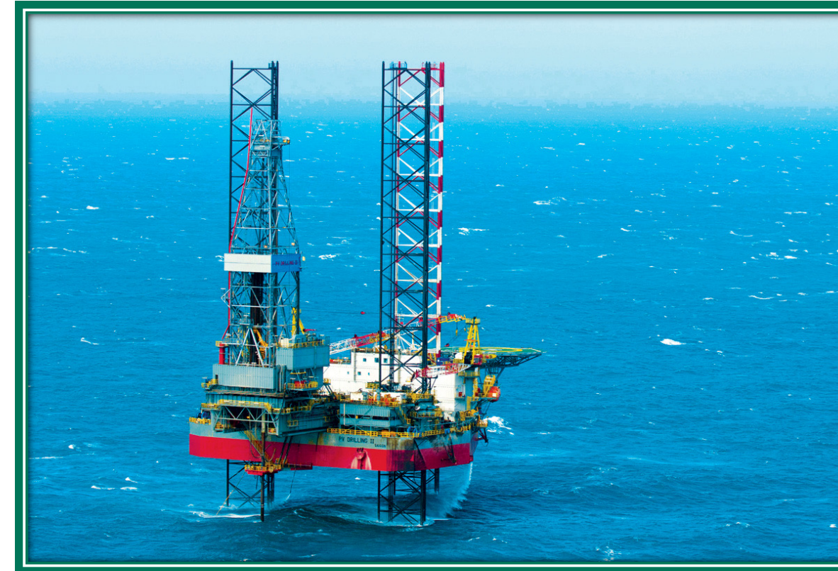
PV DRILLING II
