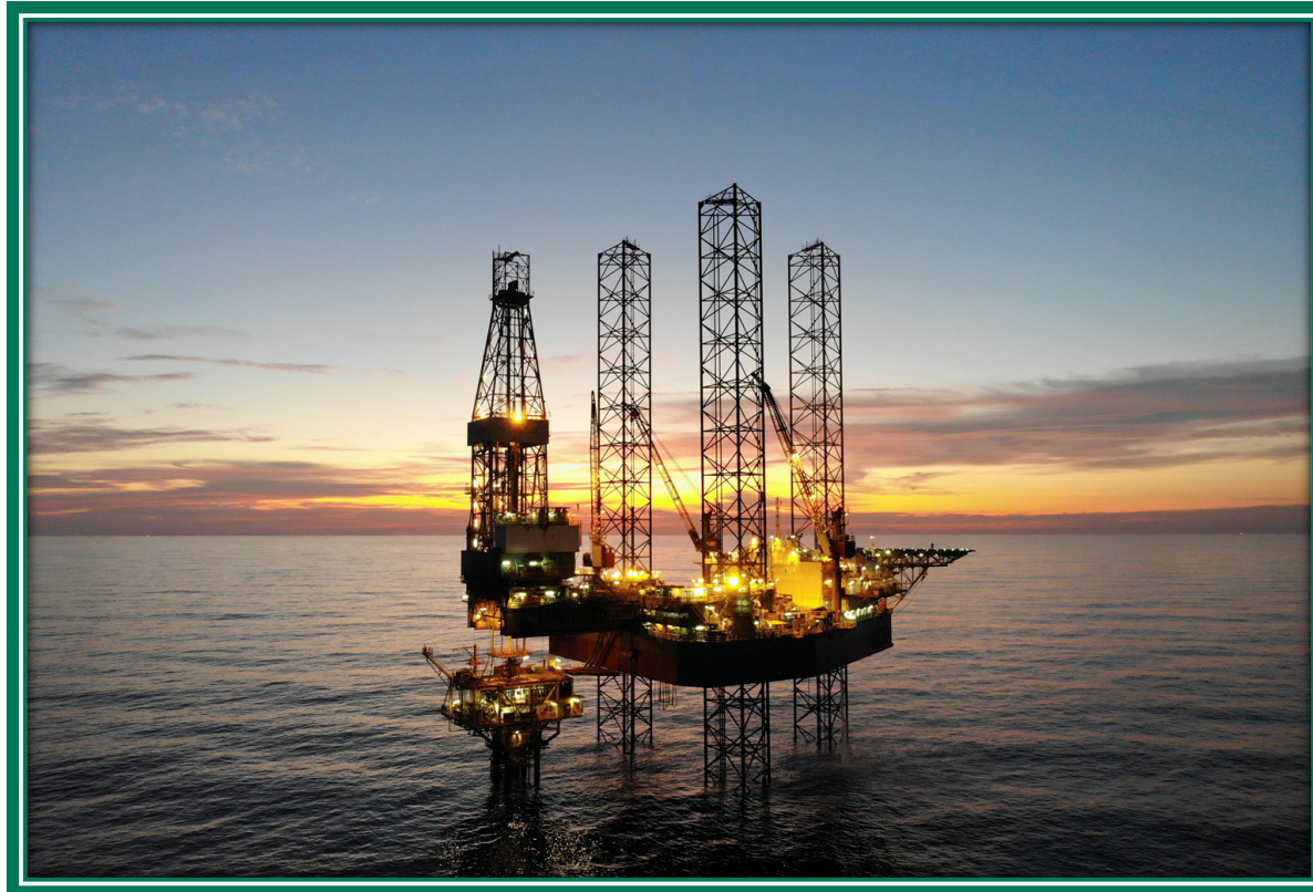
PV DRILLING I
