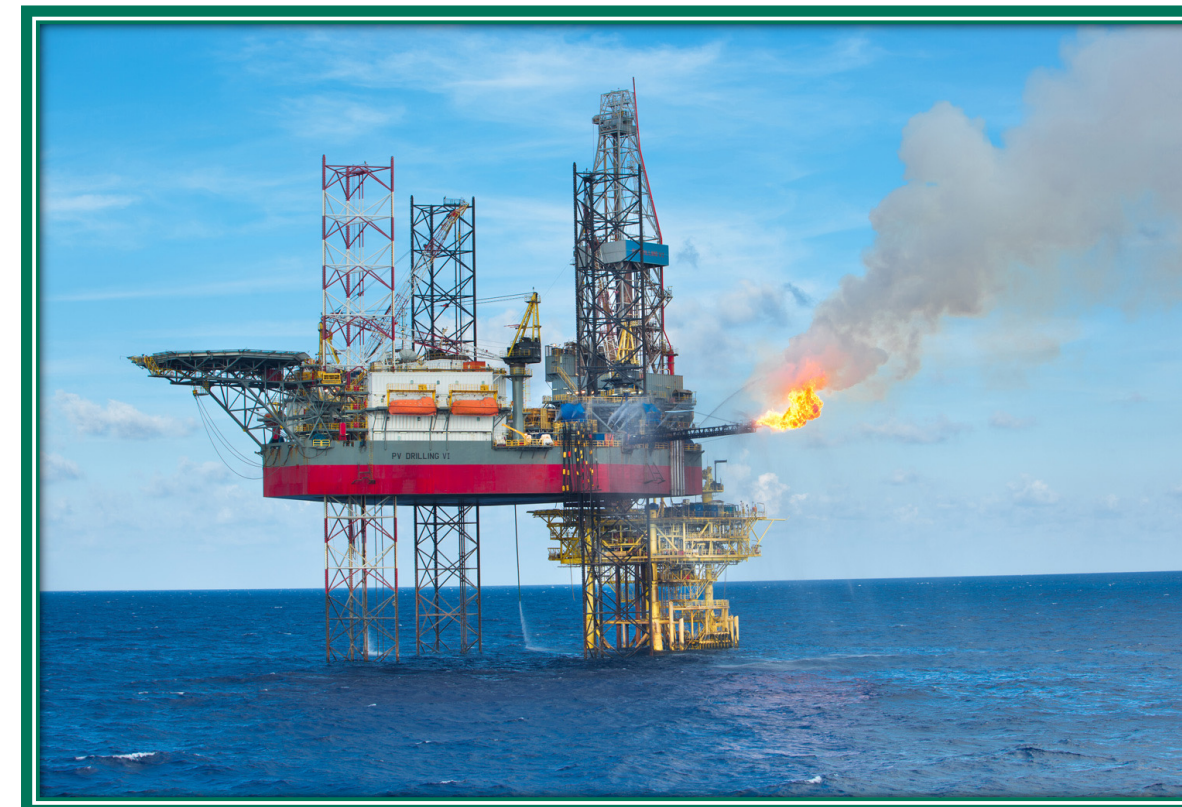
PV DRILLING V
