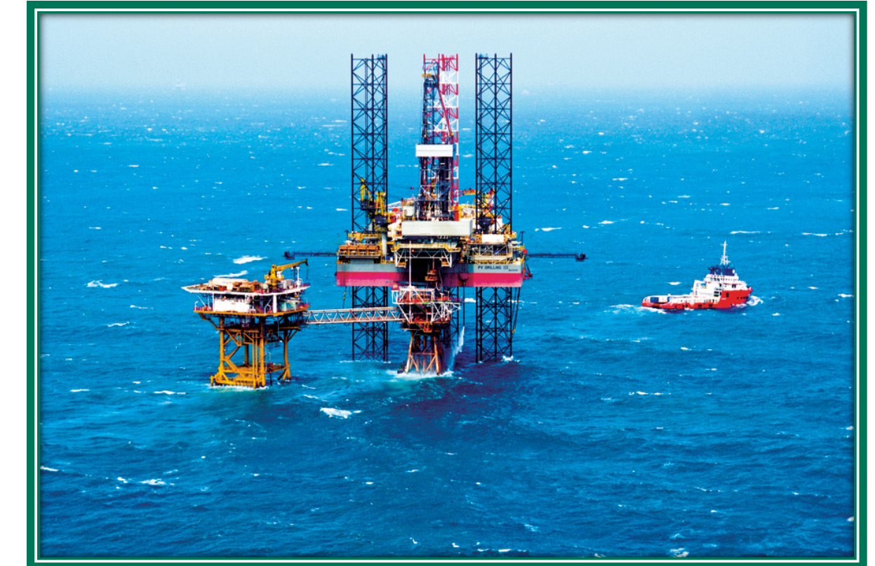
PV DRILLING III
